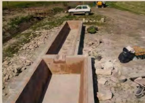
Coccio-pesto plaster used for internal lining of the basins
